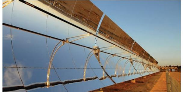
Solel's solar thermal parabolic trough technology will be used to deliver 553 MW of solar power to PG&E's customers once constructed in California's Mojave Desert.
