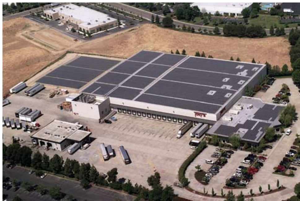
Located in West Sacramento, Tony's Fine Foods features the largest privately owned solar power system in northern California.
